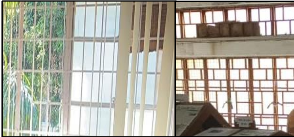
Natural Lighting facilities observed during day time
